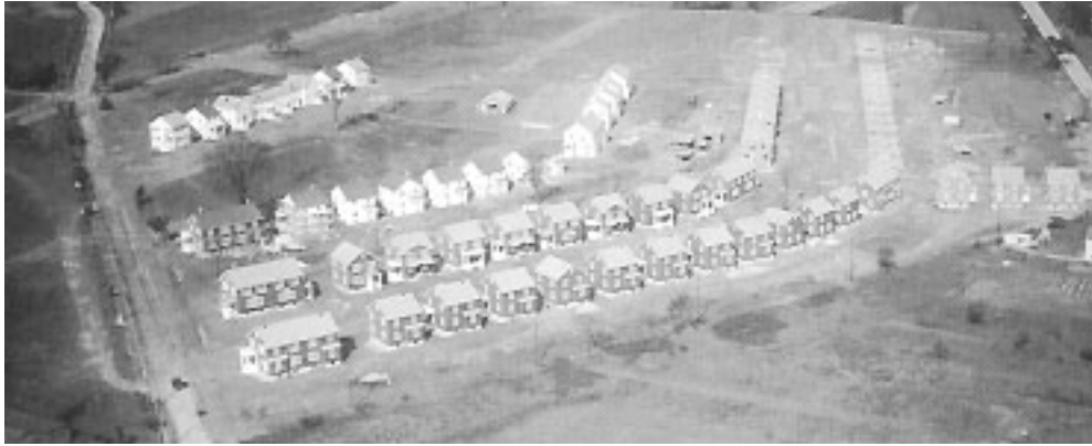
Figure 9. Garden Homes during construction. (Milwaukee County Historical Society)
