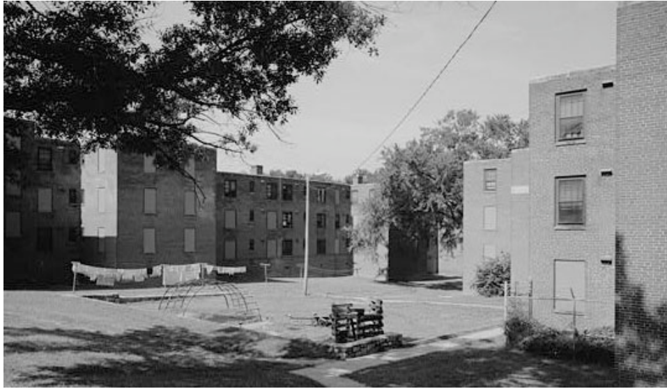
Figure 5. Techwood Homes courtyard shortly before demolition. (Library of Congress, Prints and Photographs Division, Historic American Buildings Survey or Historic American Engineering Record, HABS, GA,61-ATLA,60E-15)
