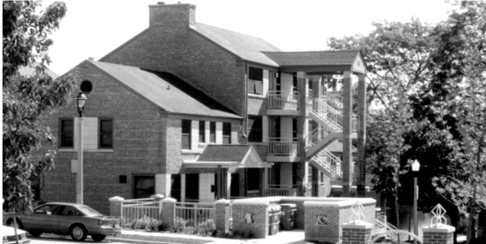
Figure 28. Fire escape and porches added as part of HOPE VI revitalization. (Courtesy of HACM)
