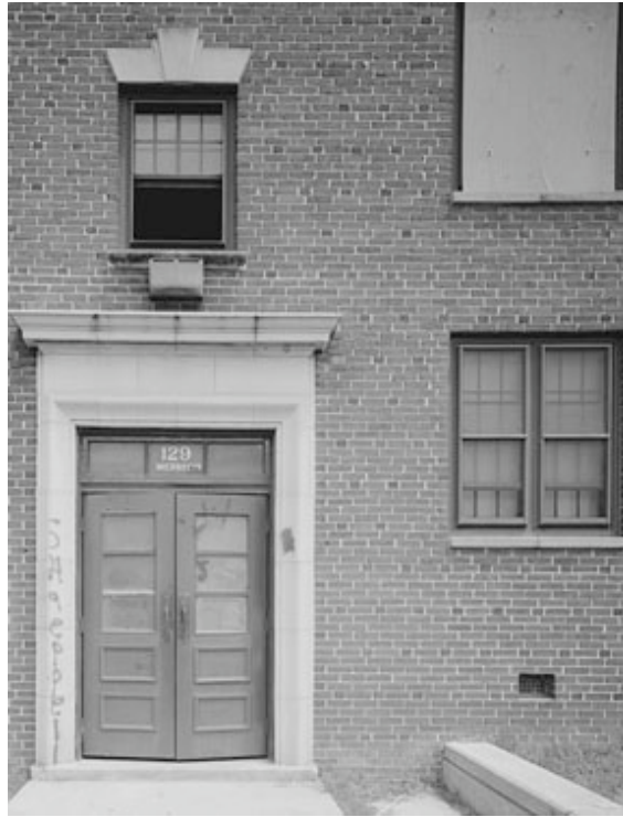
Figure 4. Entrance and window details at Techwood Homes shortly before demolition. (Library of Congress, Prints and Photographs Division, Historic American Buildings Survey or Historic American Engineering Record, HABS, GA,61-ATLA,60E-10)
