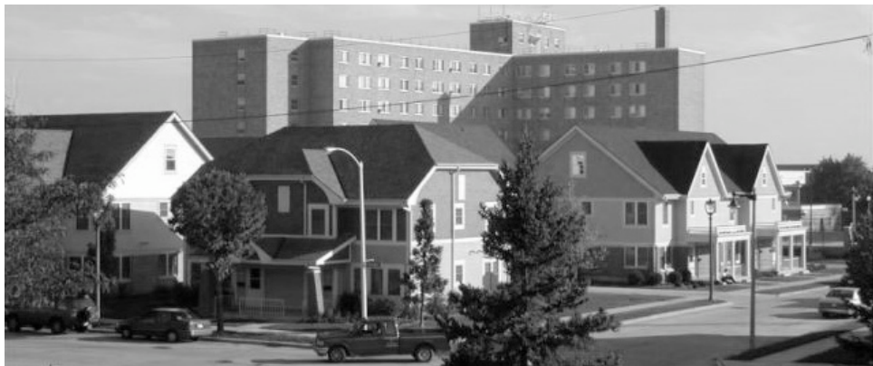
Figure 44. Lapham Park before demolition and its HOPE VI replacement, Townhomes at Carver Park. (Courtesy of HACM)
