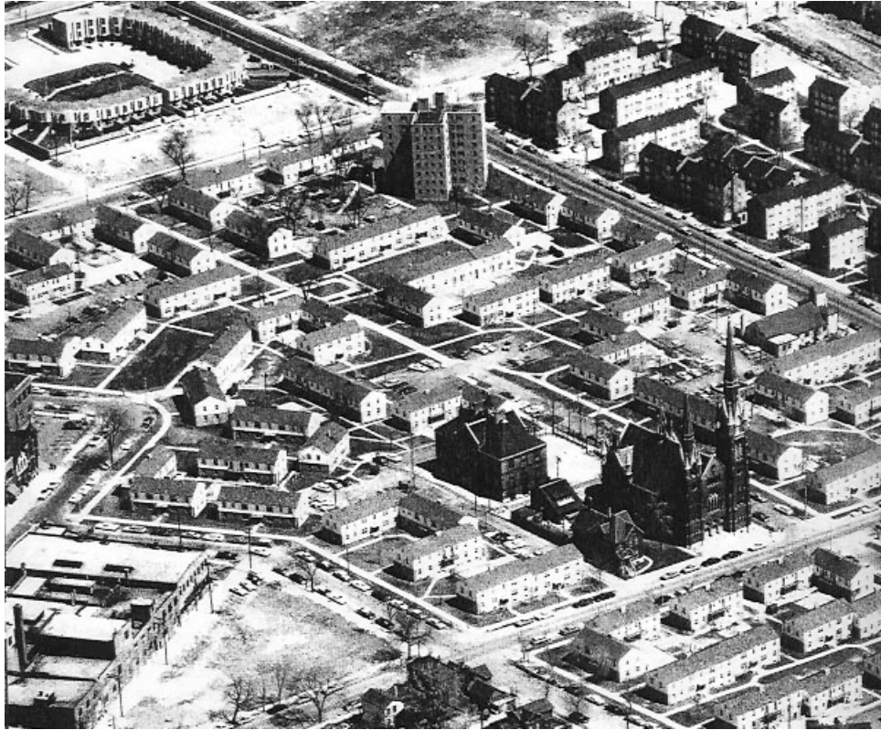
Figure 21. Hillside Terrace Addition. (Courtesy of HACM)
