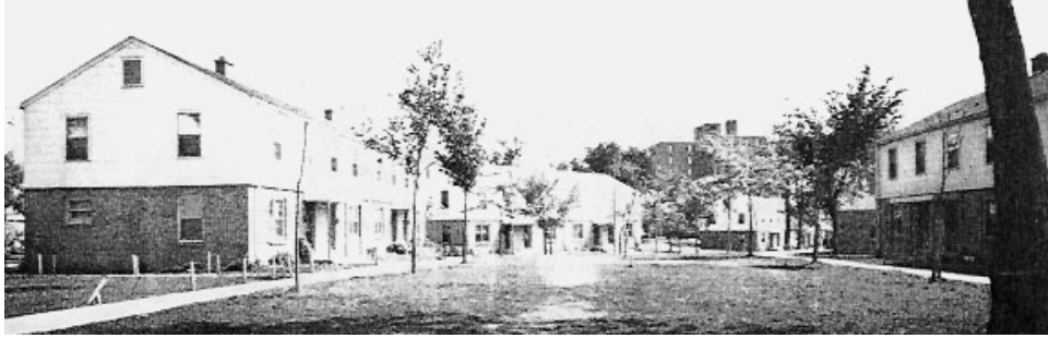
Figure 22. Hillside Terrace Addition. (Courtesy of HACM)
