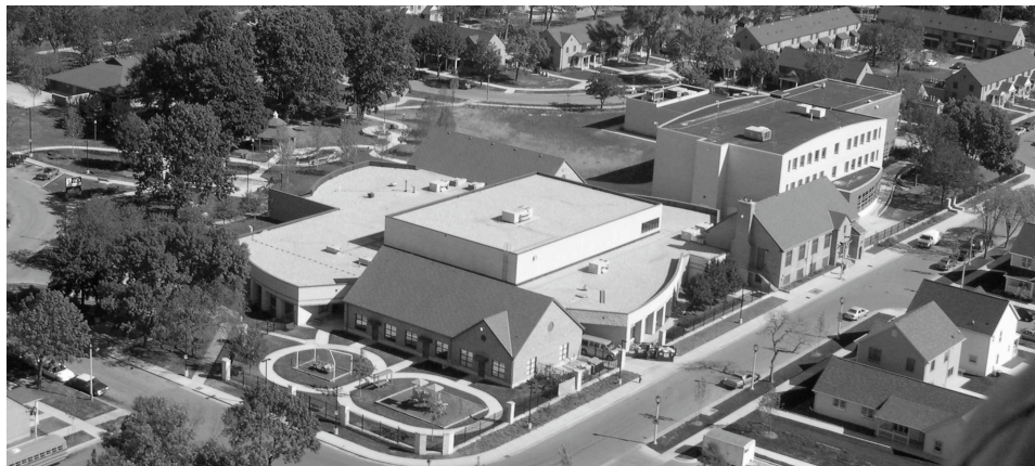
Figure 37. Park at Parklawn before and after HOPE VI revitalization. (Courtesy of HACM)
