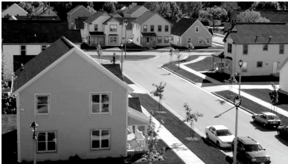
Figure 34. New homes constructed in Parklawn. (Courtesy of HACM)
