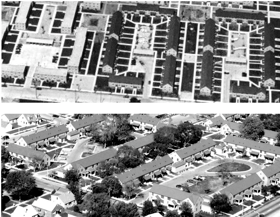
Figure 35. Parking lots at Parklawn before and after HOPE VI revitalization. (Courtesy of HACM)
