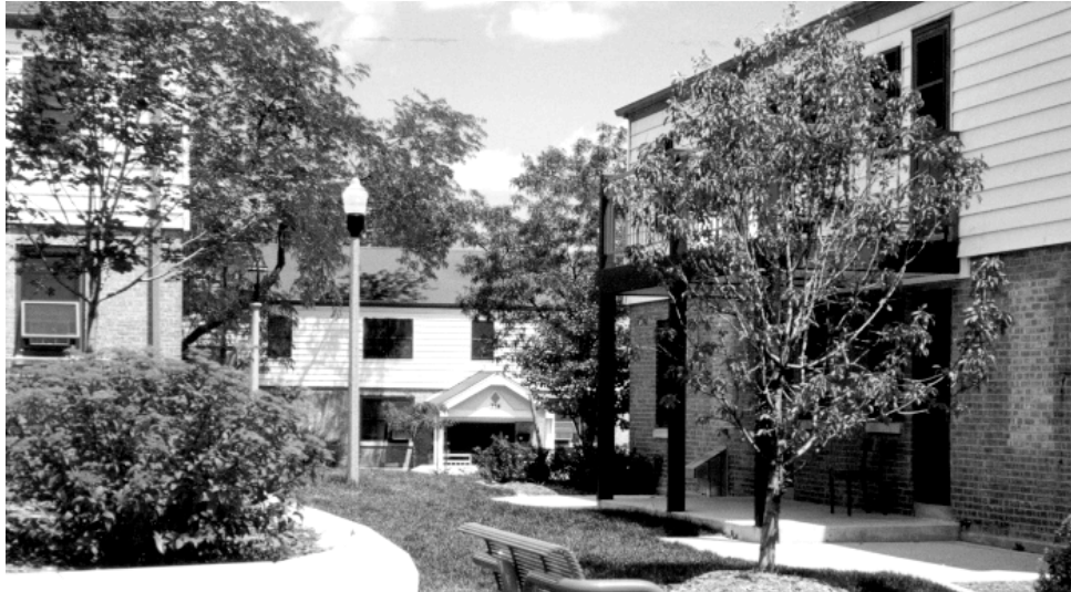
Figure 29. Front and back porches at Hillside Terrace Addition before and after HOPE VI revitalization. (Courtesy of HACM)
