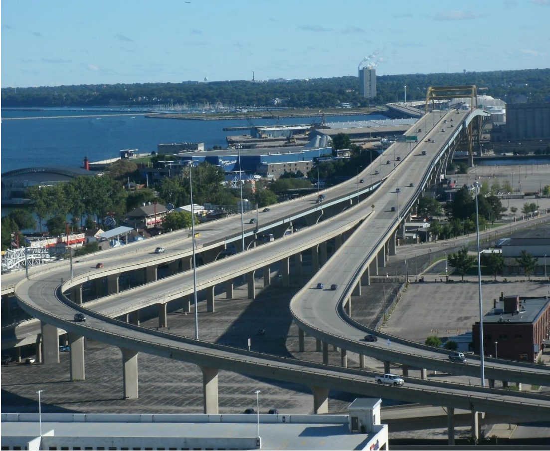
Figure 9: The Lake Interchange and I-794, facing south. Photo by Greg Dickenson, 2013.
