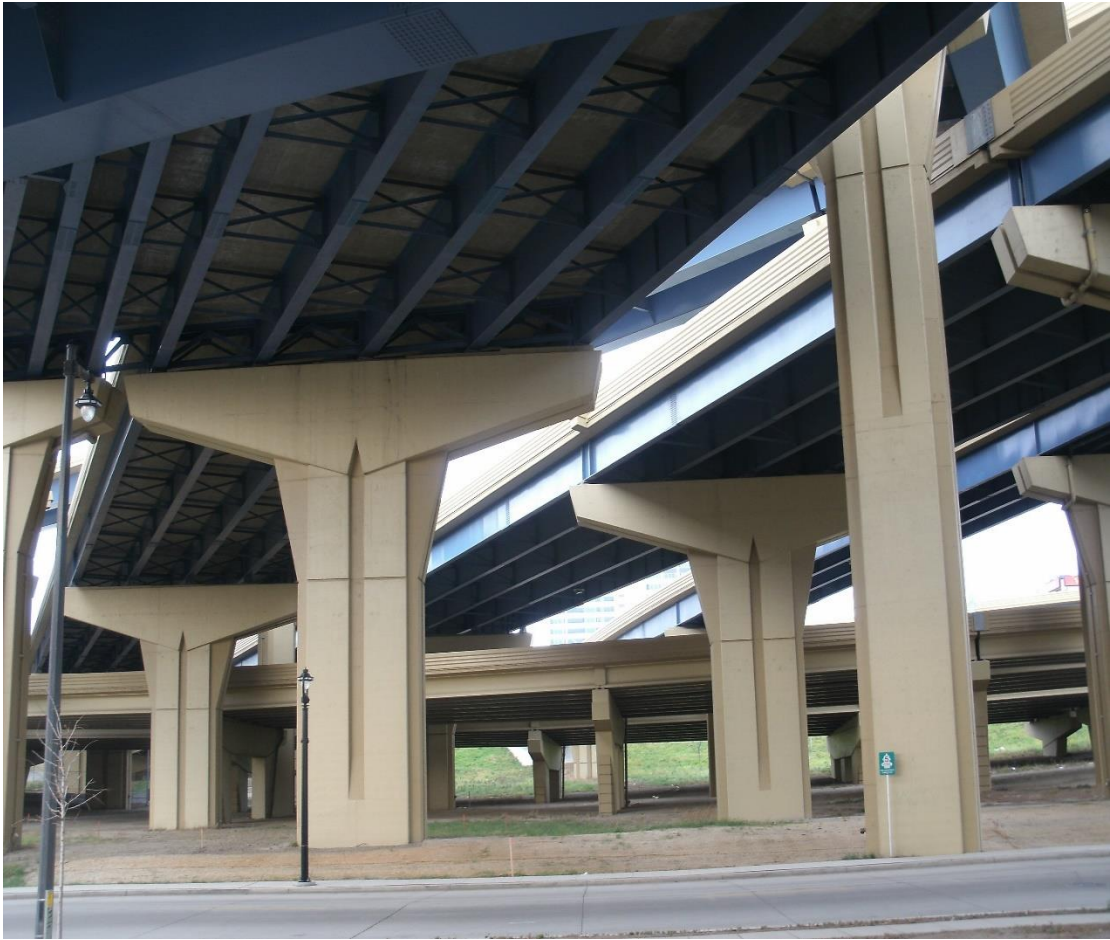
Figure 8: This is a view along West St. Paul Avenue under the Marquette Interchange. Photo by Greg Dickenson, 2012.
