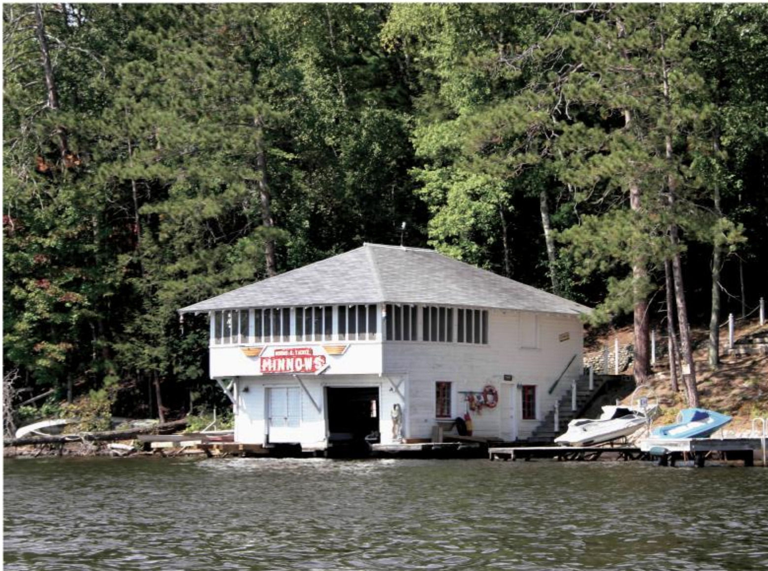
Two-slip, two-story boathouse on the Three Lakes chain of lakes
