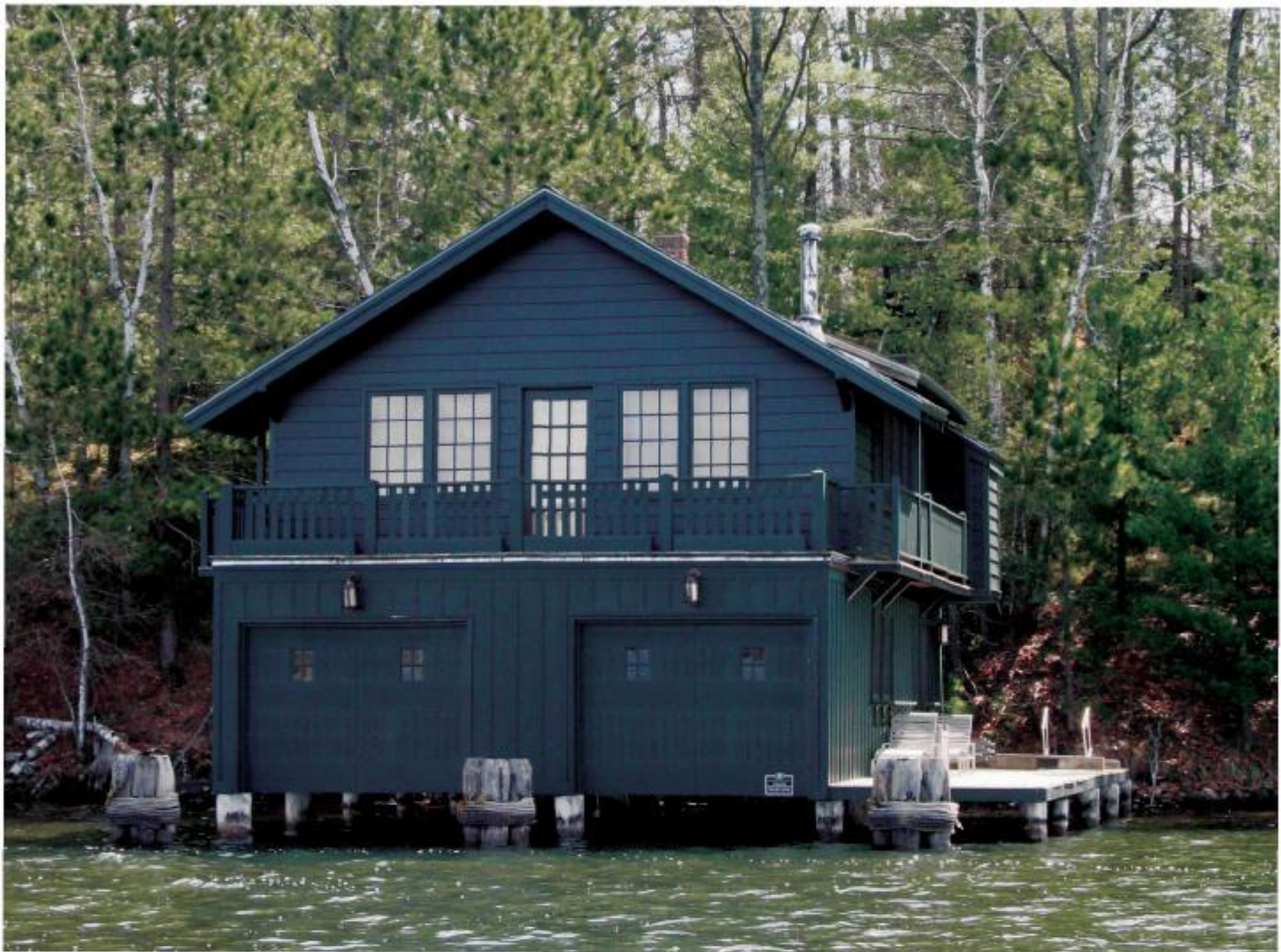
The Craftsman-style Ella M. Boesel boathouse on Lake Minocqua was built ca.1935. It was the first boathouse to be individually listed in the National Register of Historic Places.
